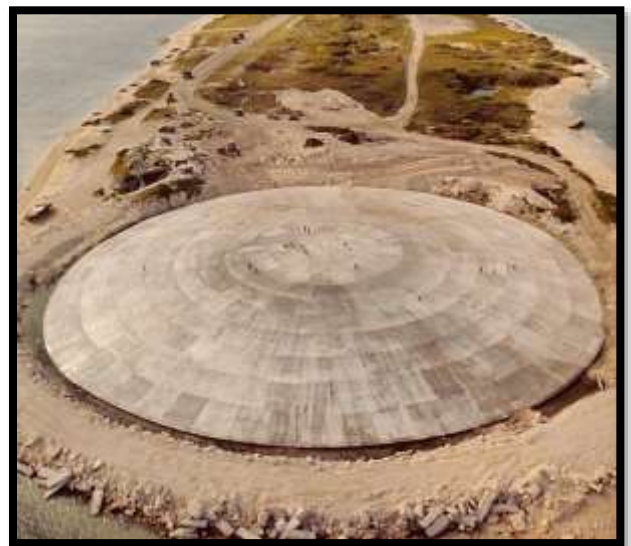
Figure 3 Runit Dome in the Marshall Islands. The dome encases radioactive waste from nuclear test explosions. Wikimedia Commons image.
