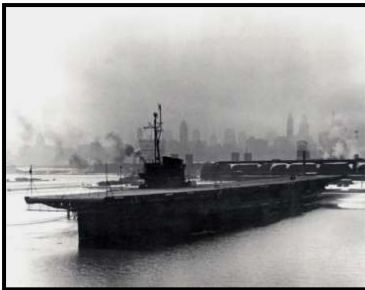
Figure 4 USS Sable moored at Chicago's Navy Pier during WWII (Courtesy, Naval History and Heritage Command).
