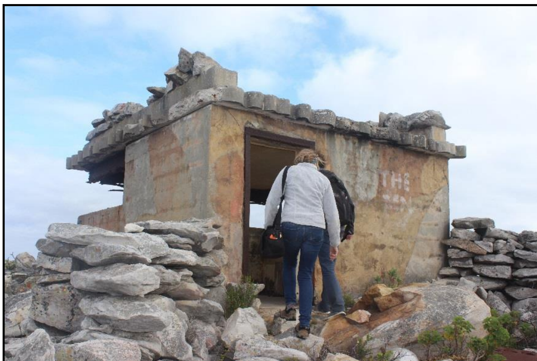
Figure 23. Bosch Radar Observation Structure. Note the camouflage techniques with rocks around the structure and on the roof (ECU Photograph).
